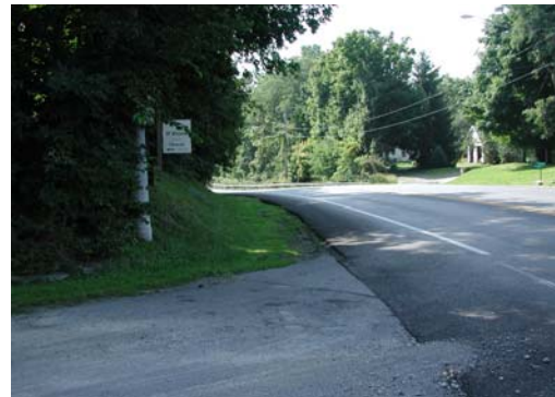
Intersection of Route 15 @ Railroad Ave. – Sight distance obstruction
