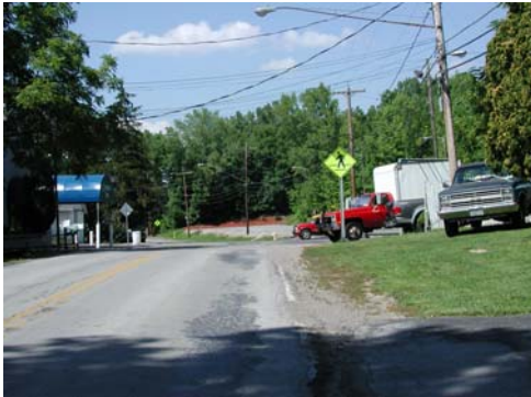
East Lake Road near Conesus Inn – poor pavement edge
