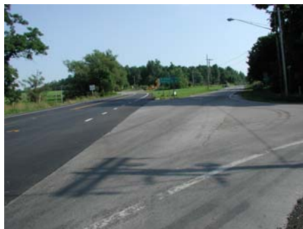
East Lake Road near Leisure Marina – undefined pavement edge
