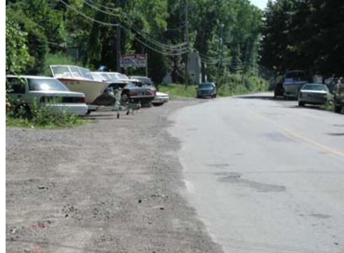
East Lake Road near Leisure Marina – undefined pavement edge
