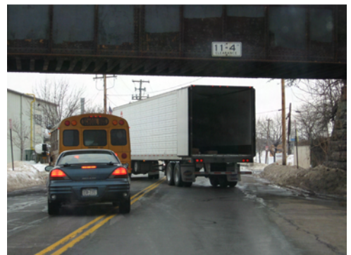
Substandard Vertical Clearance
