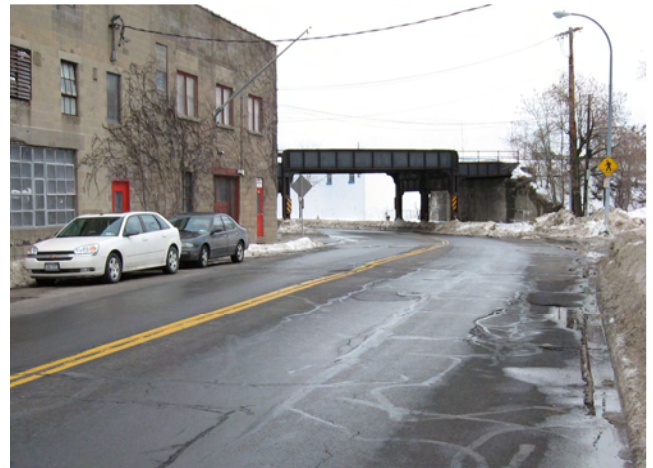
Substandard Stopping Sight Distance
