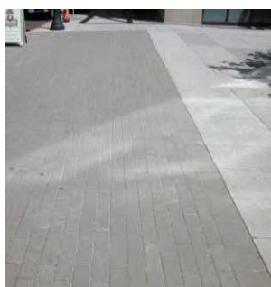
Concrete Unit Pavers
