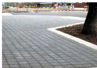
Concrete Unit Pavers
