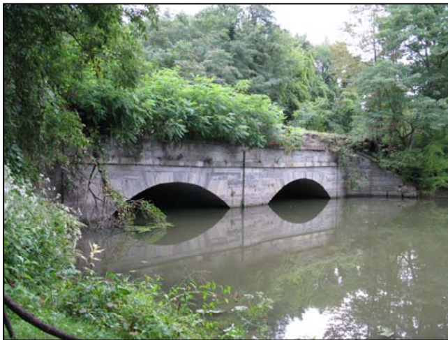
The double-arched stone culvert at Black Creek is one of the largest culverts constructed on the nineteenth century New York State Canal System.
