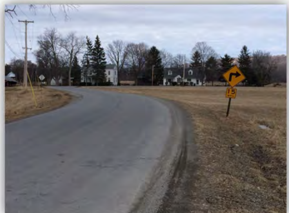
Geometric constraints at Meter and Zerfass Road intersection not suitable to handle a projected increase in traffic volume from future development.
