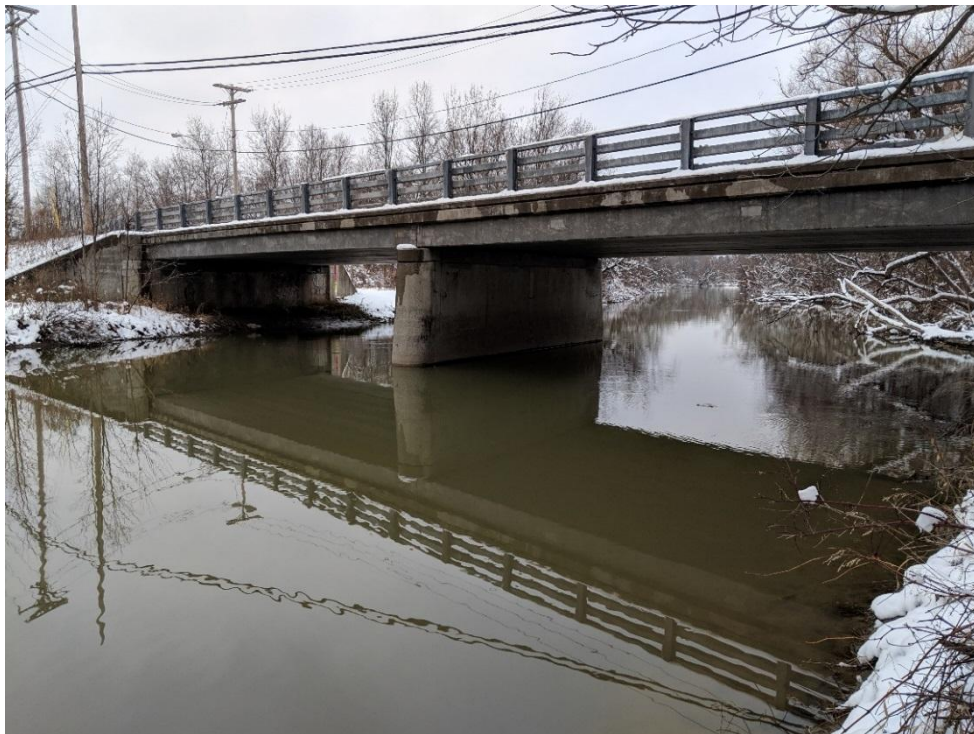
(looking north, upstream side): Two-span adjacent prestressed concrete box beams.
