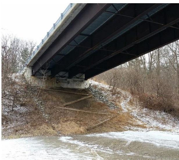
(looking northwest): Steel stringers and girders. Slope stabilization.
