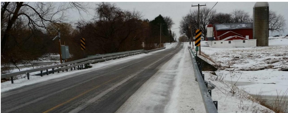
(looking east): BIN 3317640– asphalt wearing surface on cast-in-place concrete deck.
