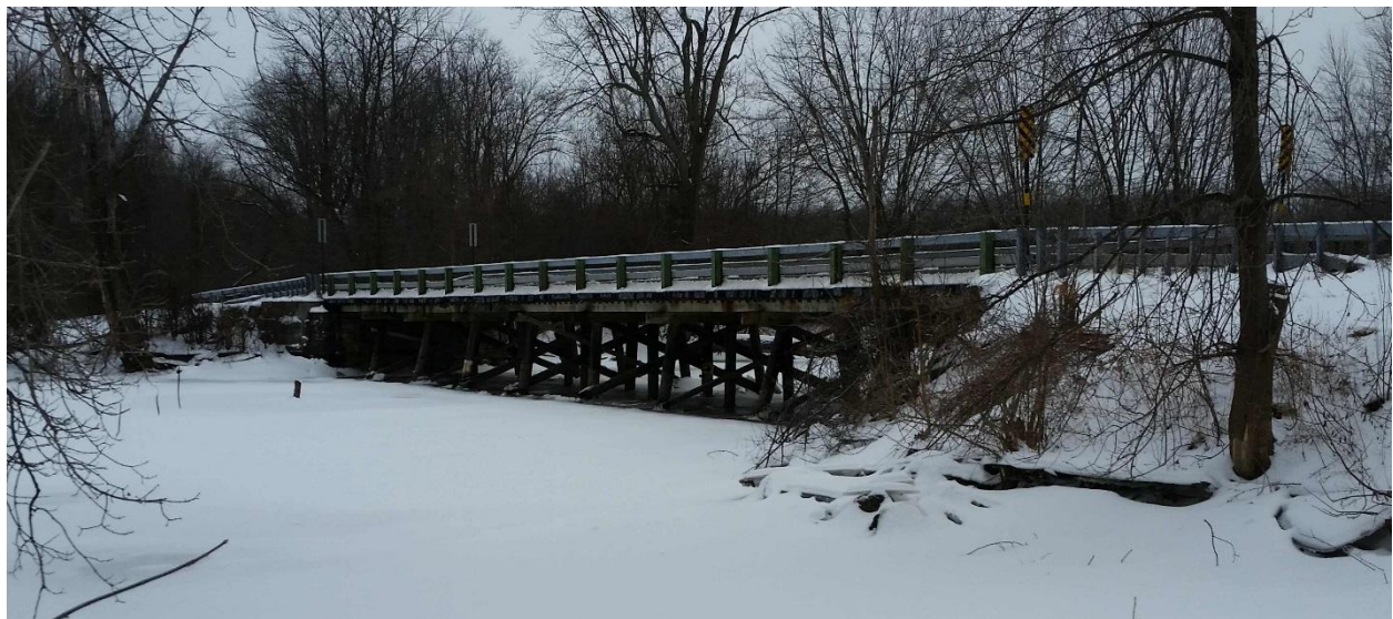
(looking south, downstream side): Wooden timber multi-span bridge on wooden pile bents.
