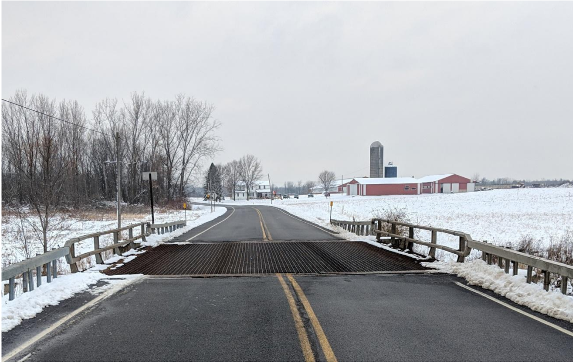
(looking north): BIN 3315450 – Open steel grid deck.
