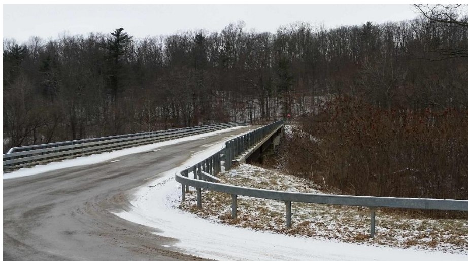
(looking northwest): BIN 3319860 – asphalt wearing surface on stay-in-place formed concrete deck.
