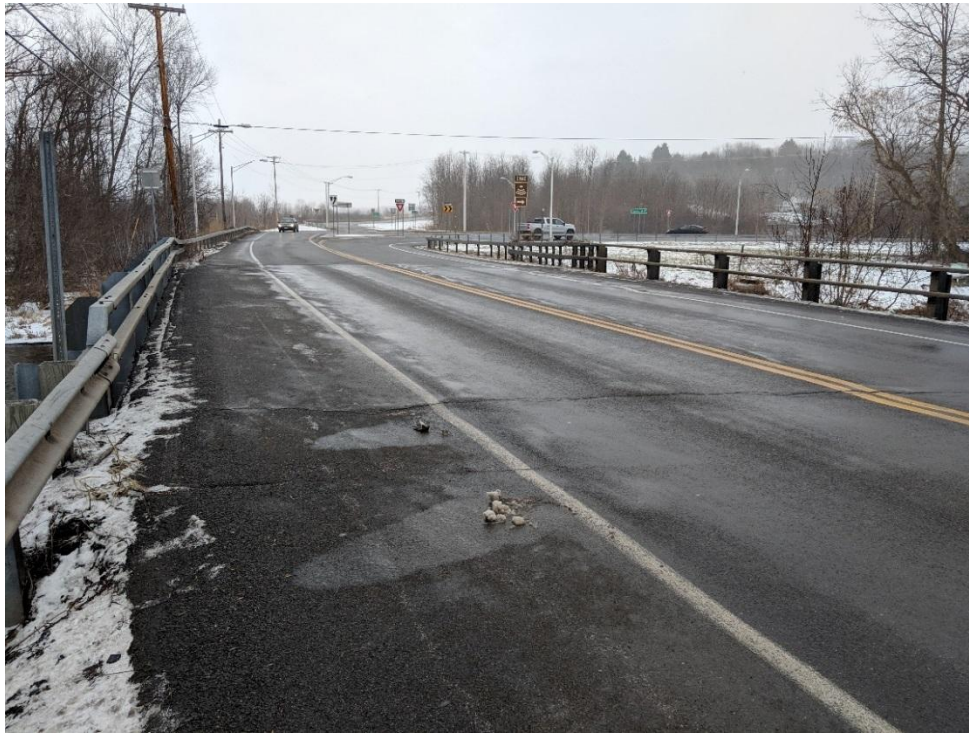
(looking east): BIN 3318660 – Asphalt wearing surface on adjacent box beams.
