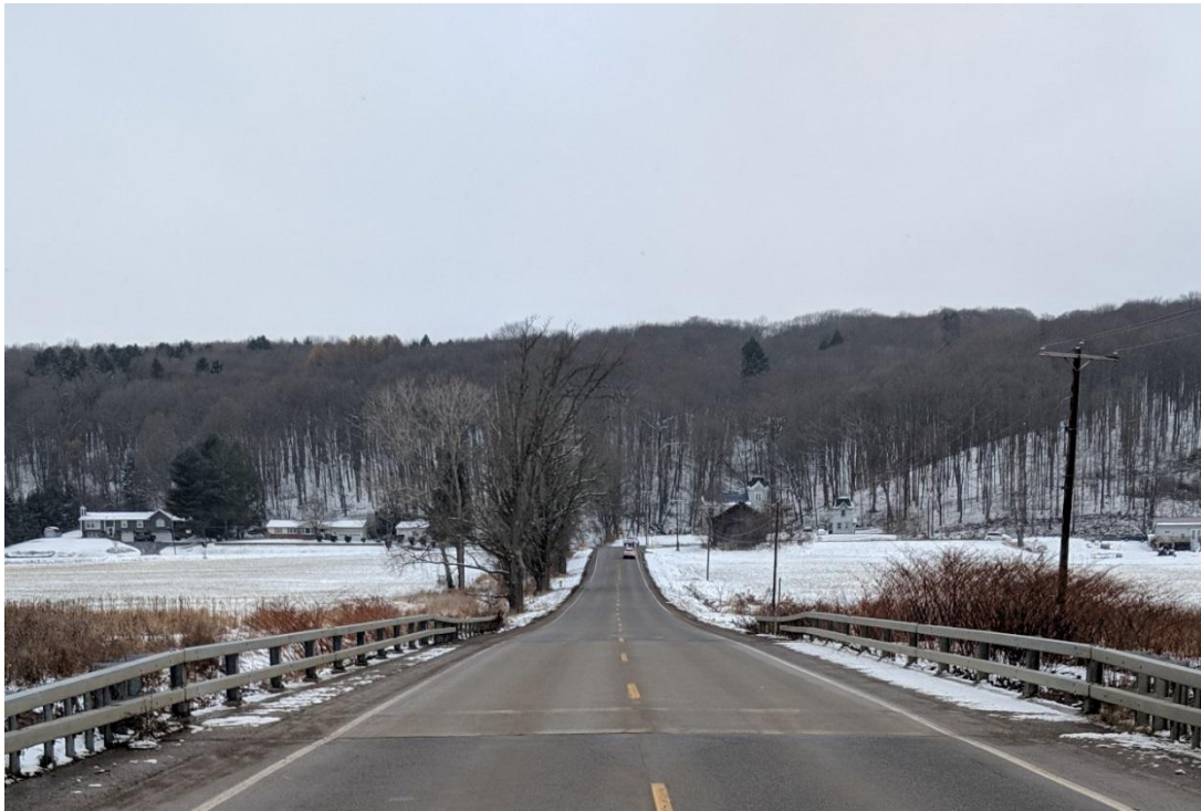
(looking west): BIN 3366430 – Monolithic Concrete deck on adjacent box beams.
