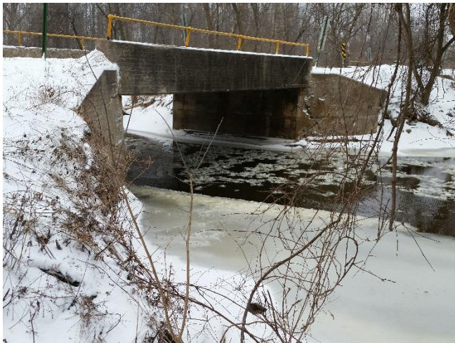
(looking south, upstream side): concrete abutments and wingwalls, constriction of flow.
