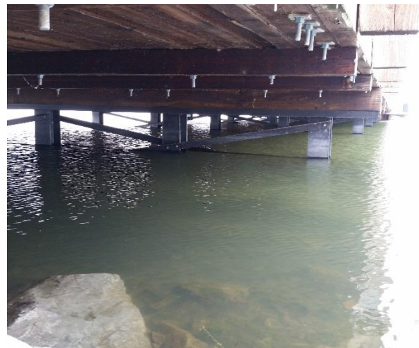
(looking east, upstream side): Wood/timber multi-span deck supported on steel H-pile bents.
