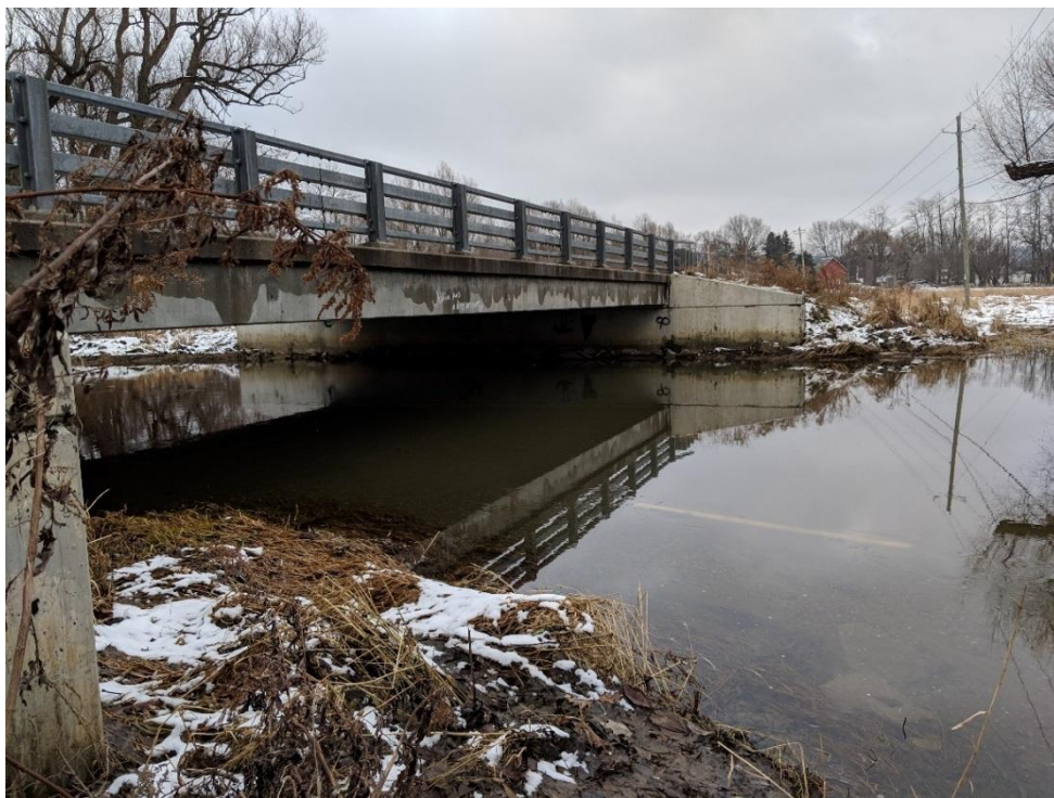
(looking east, upstream side): Single span adjacent prestressed concrete box beams.
