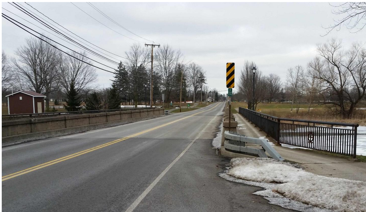
(looking north): BIN 3317290– asphalt wearing surface on cast-in-place concrete deck.
