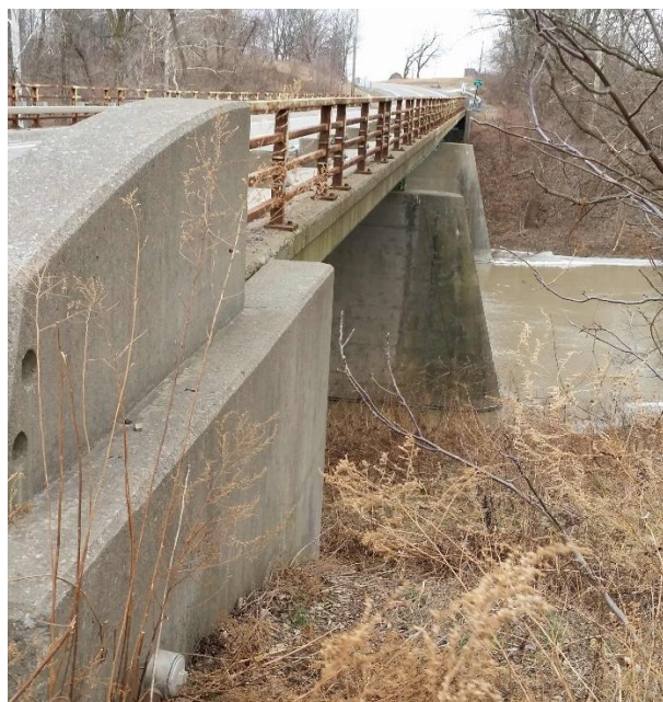
(looking east, upstream side): Three-span bridge with two solid wall concrete piers and concrete abutments.
