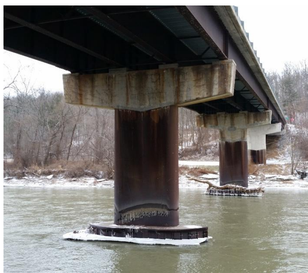
(looking northwest, downstream side): Four-span bridge with three armored, hammerhead concrete piers and concrete abutments. Debris in channel, erosion of banks.
