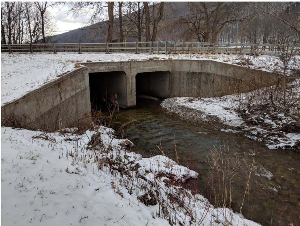
(looking northeasterly, upstream side): Double box CIP concrete culvert bridge.
