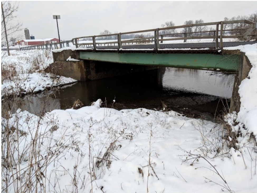
(looking east, downstream side): Single span steel multi-girder bridge.
