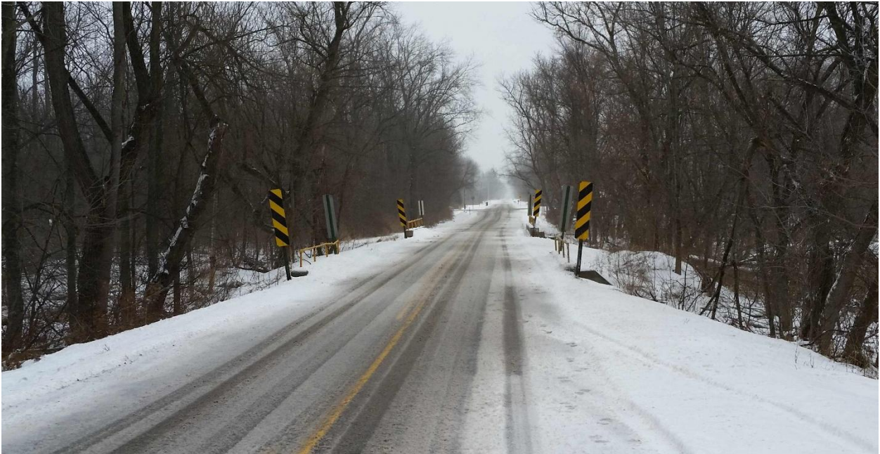
(looking north): BIN 3319170 – asphalt wearing surface on concrete deck (note the sub-standard guide rail protection).
