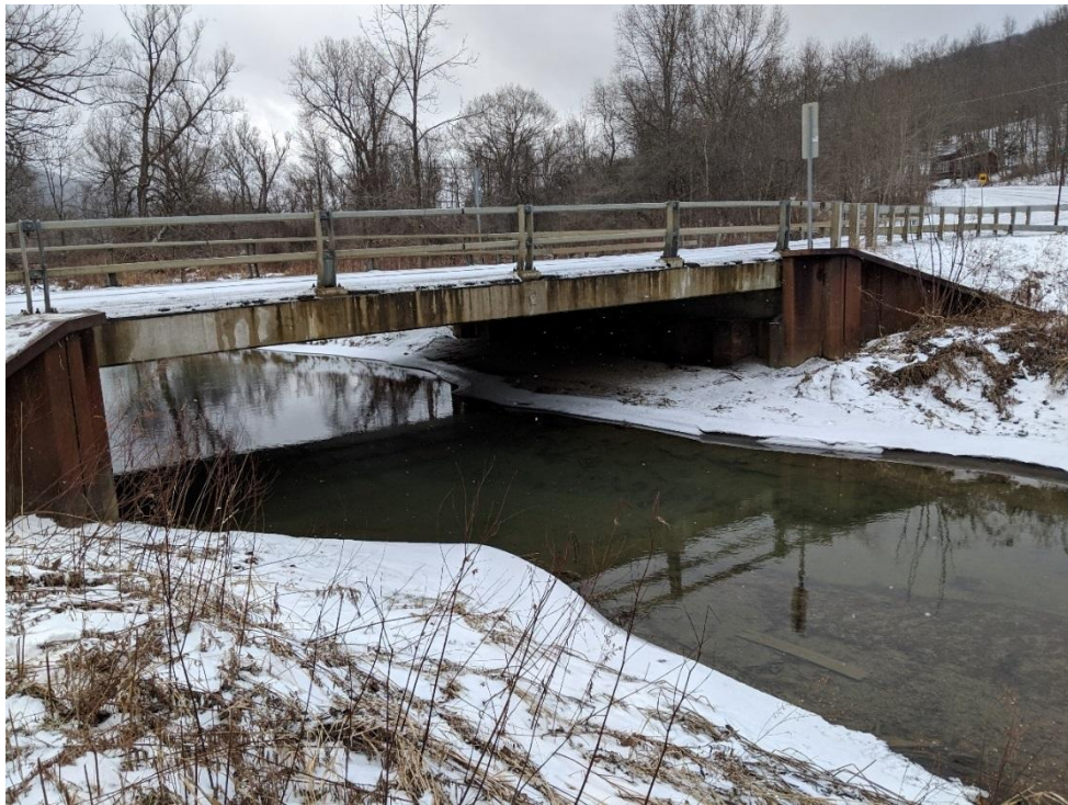
(looking south, downstream side): Single span adjacent prestressed concrete box beams.
