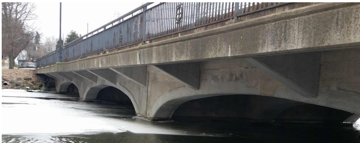
(looking south, downstream side): Concrete superstructure, cantilevered sidewalk, and concrete substructure.
