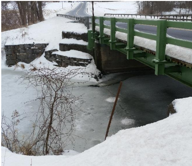
(looking east, downstream side): Some wingwall stones have fallen into the creek.
