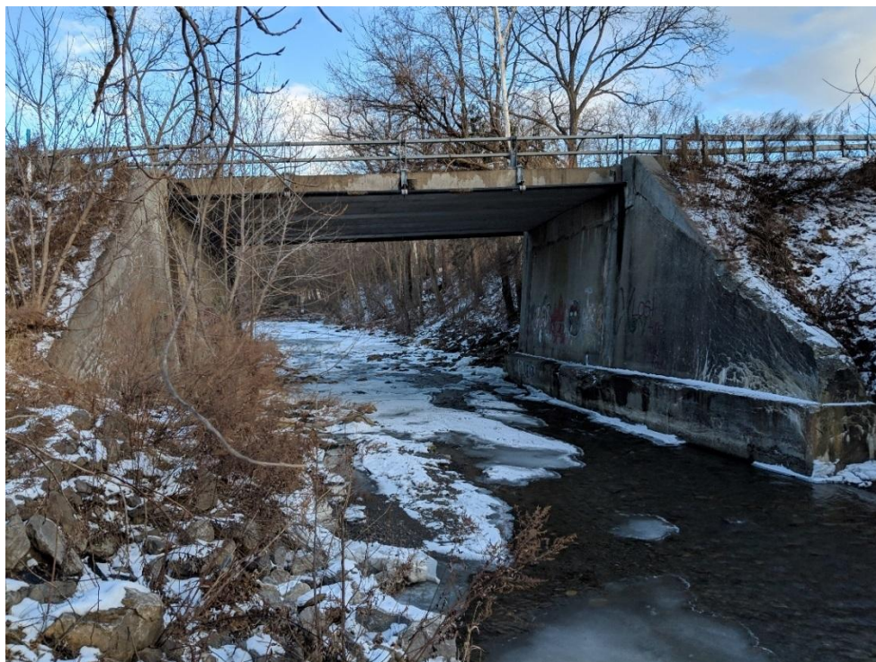
(looking east, downstream side): Single span adjacent prestressed concrete box beams.
