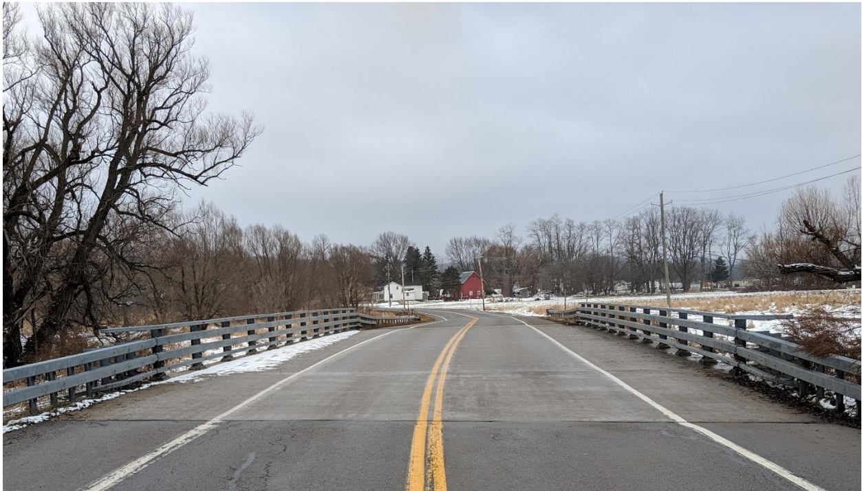
(looking south): BIN 3319950 – Monolithic Concrete deck on adjacent box beams.
