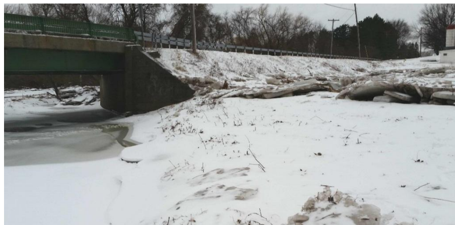
(looking north, downstream side): Evidence of ice jamming downstream (north east) of bridge.
