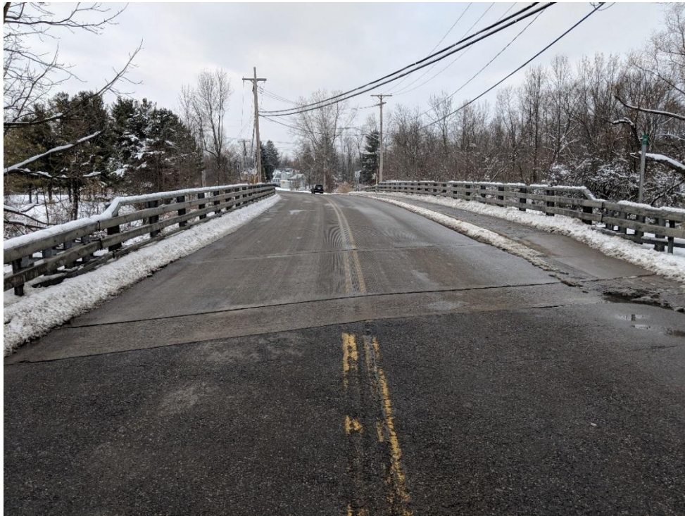
(looking west): BIN 2210840 – Monolithic concrete deck and sidewalk.
