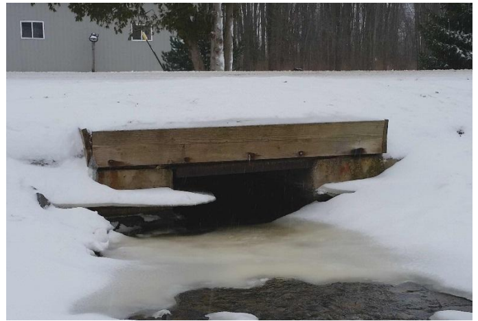
(looking east, upstream side): bank erosion, debris in channel, and evidence of ice jamming.
