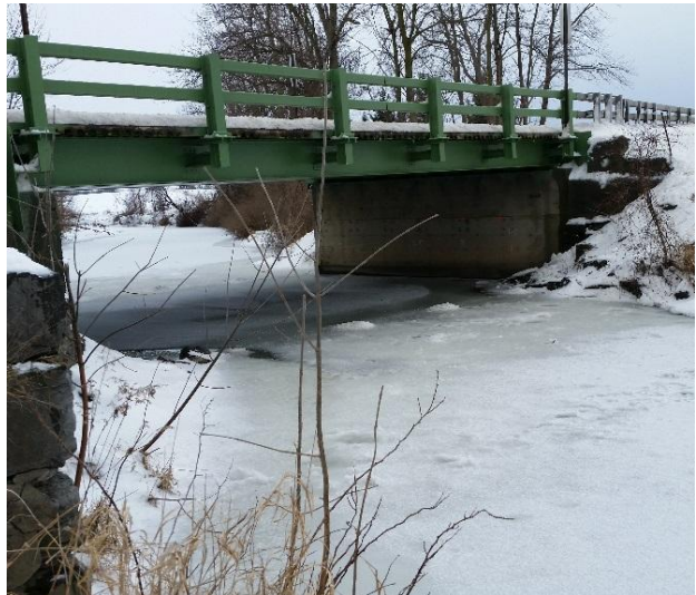
(looking west, downstream side): Some wingwall stones have fallen into the creek.
