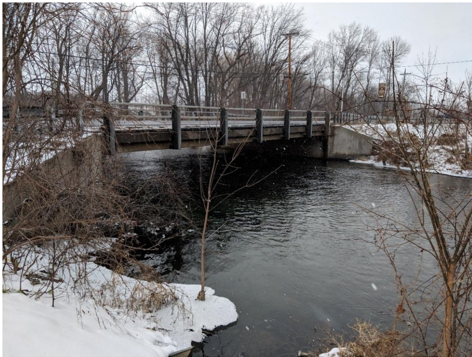
(looking north, upstream side): Single span adjacent prestressed concrete box beams.
