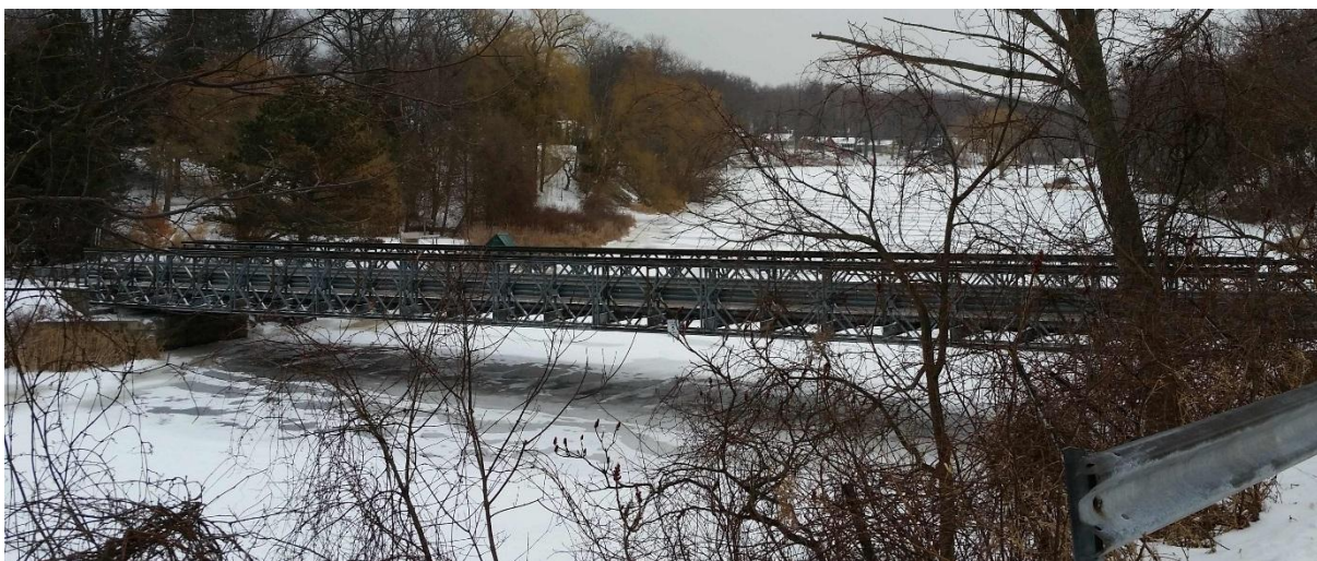
(looking east, downstream side): Steel superstructure carried by concrete abutments.
