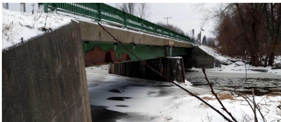
(looking west, upstream side): Steel superstructure carried by concrete pier and abutments.
