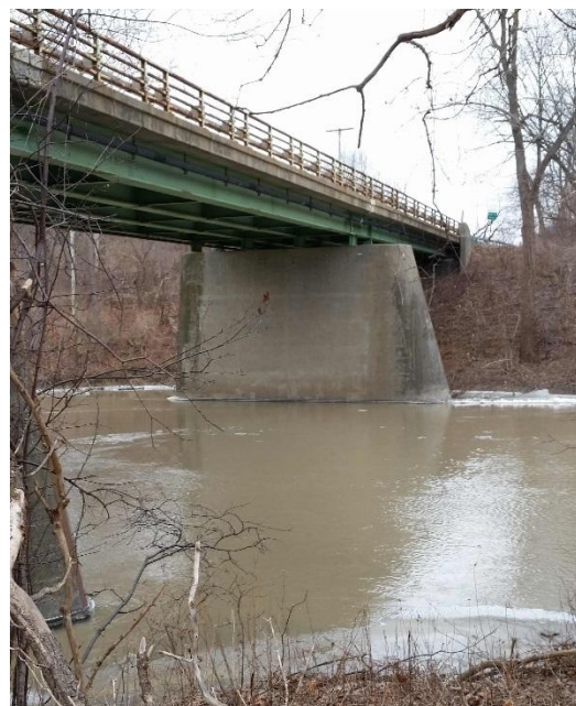
(looking east, upstream side): Steel stringers and girders.
