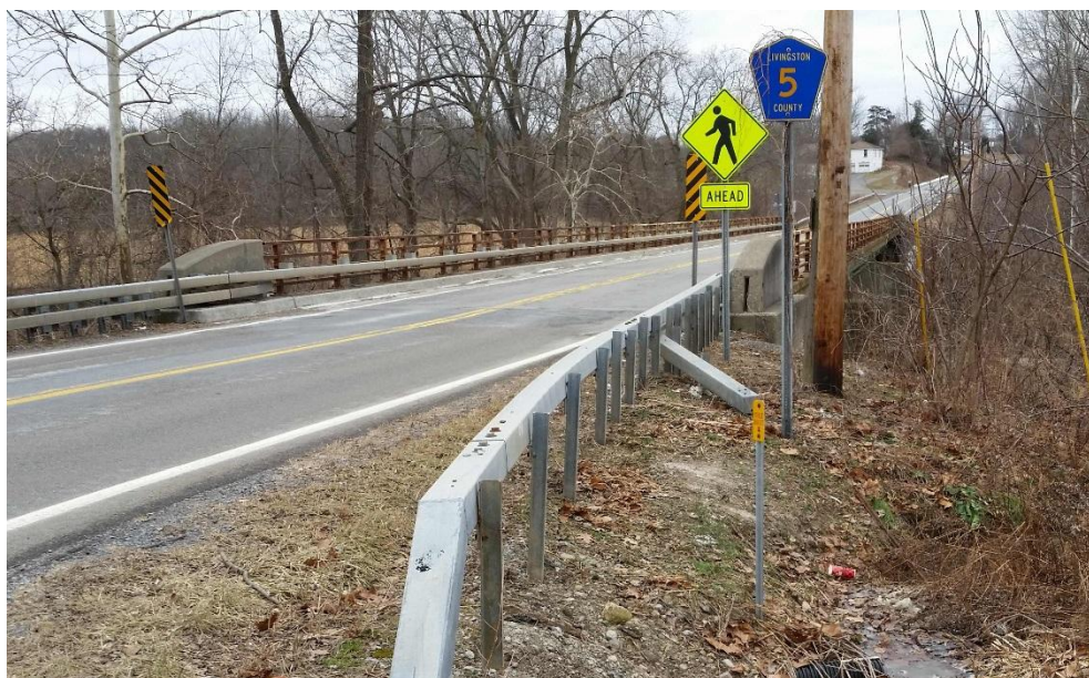
(looking west): BIN 3316240 – asphalt wearing surface on cast-in-place concrete deck.
