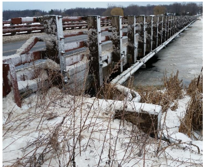
(looking east, upstream side): Utilities (Cable TV, Electric – RG&E) carried by bridge.
