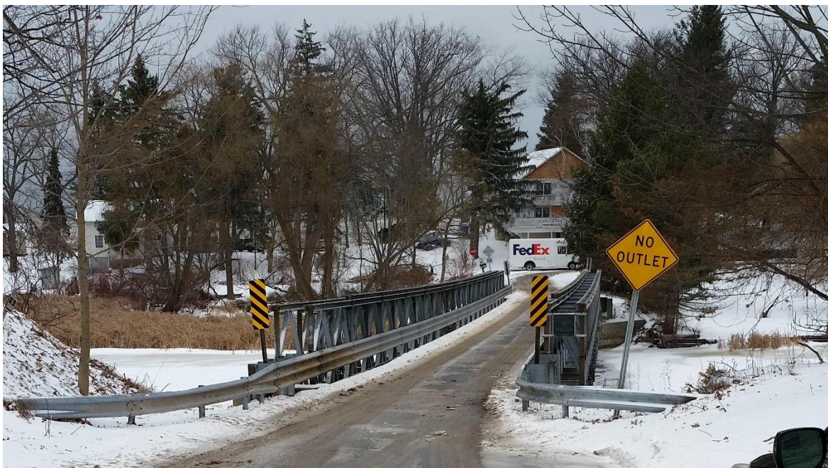
(looking north): BIN 3318990 – Galvanized steel thru-truss (Bailey bridge).
