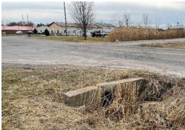
Damaged headwall along Dean Parkway
