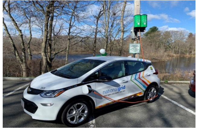
Figure 4.4: Streetlight EVSE in Melrose, Massachusetts
