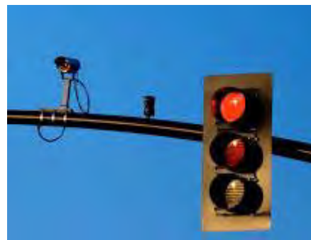
Example of Detection equipment for Adaptive Signal Control
