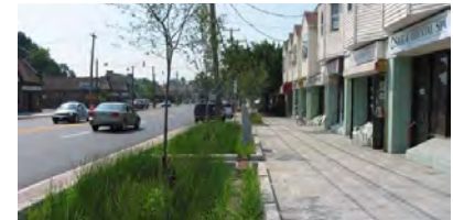
Pictured above are examples of naturalized stormwater planter systems that collect stormwater runoff.
