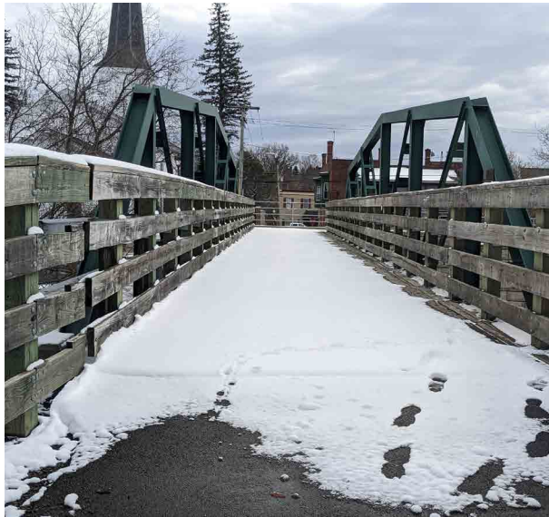
Pedestrian bridge over Cattaraugus Creek at Sanford Ave
