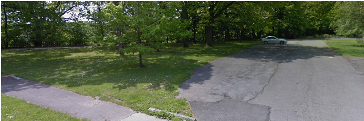
Existing Conditions at parking lot looking South
