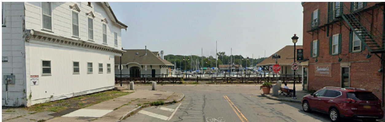
Existing Conditions of the Latta Road and River Street intersection looking East
