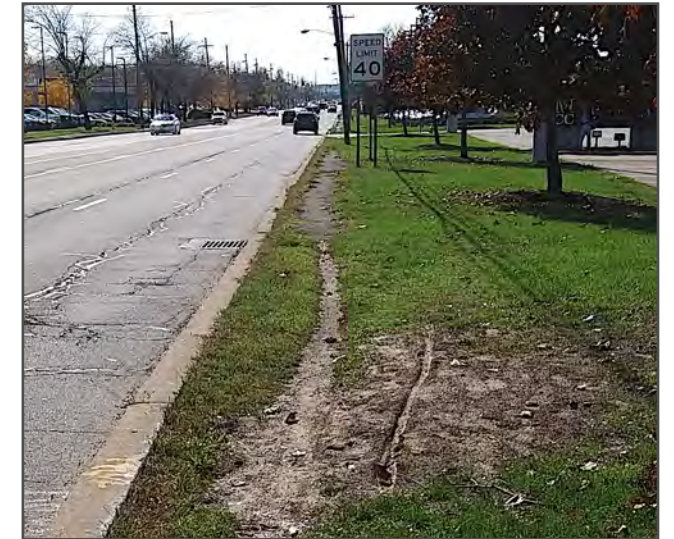
Desire paths are observed along many high-speed roadways, indicating that there is pedestrian demand despite a lack of safe facilities
