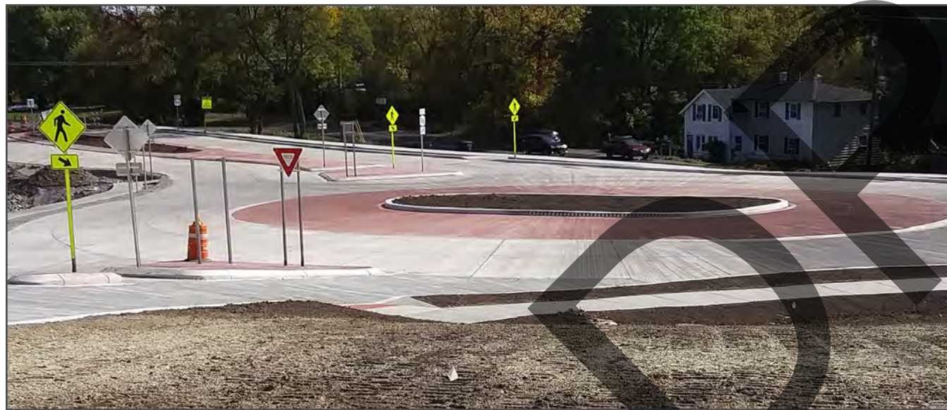
New Traffic Roundabout at New York State Route 96 and Lynaugh Road in Victor
