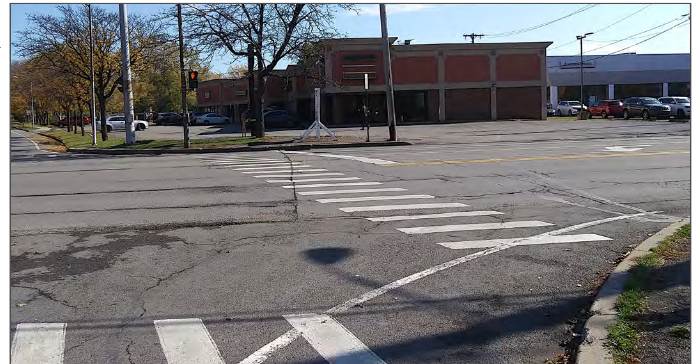
Many larger intersections have long crossing distances, but lack pedestrian safety measures such as curb cuts and refuge islands
