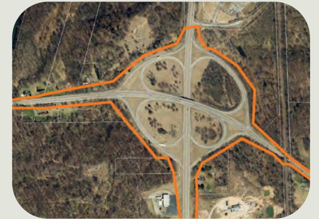
Photo: Route 96 over Route 14 Interchange Project Area
