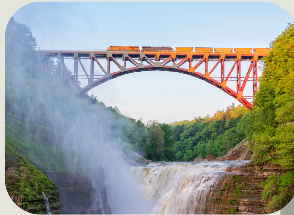
Photo: Freight Train over Letchworth Park
