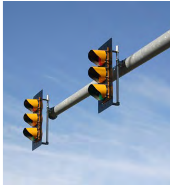
Example Signal Backplates
